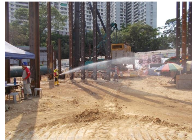
Dust suppression during breaking works
