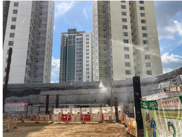
Install dust suppression sprinkler on top of hoarding
