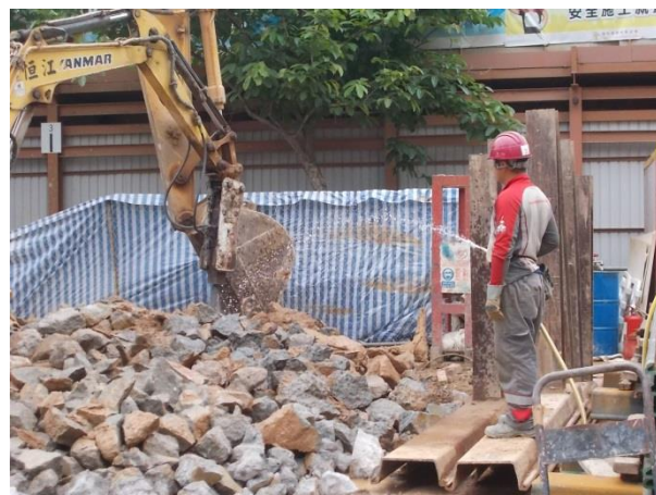
Dust suppression during breaking works
