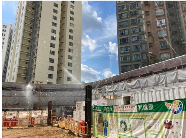
Install dust suppression sprinkler on top of hoarding
