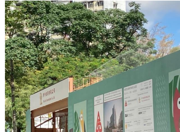
Install dust suppression sprinkler on top of hoarding
